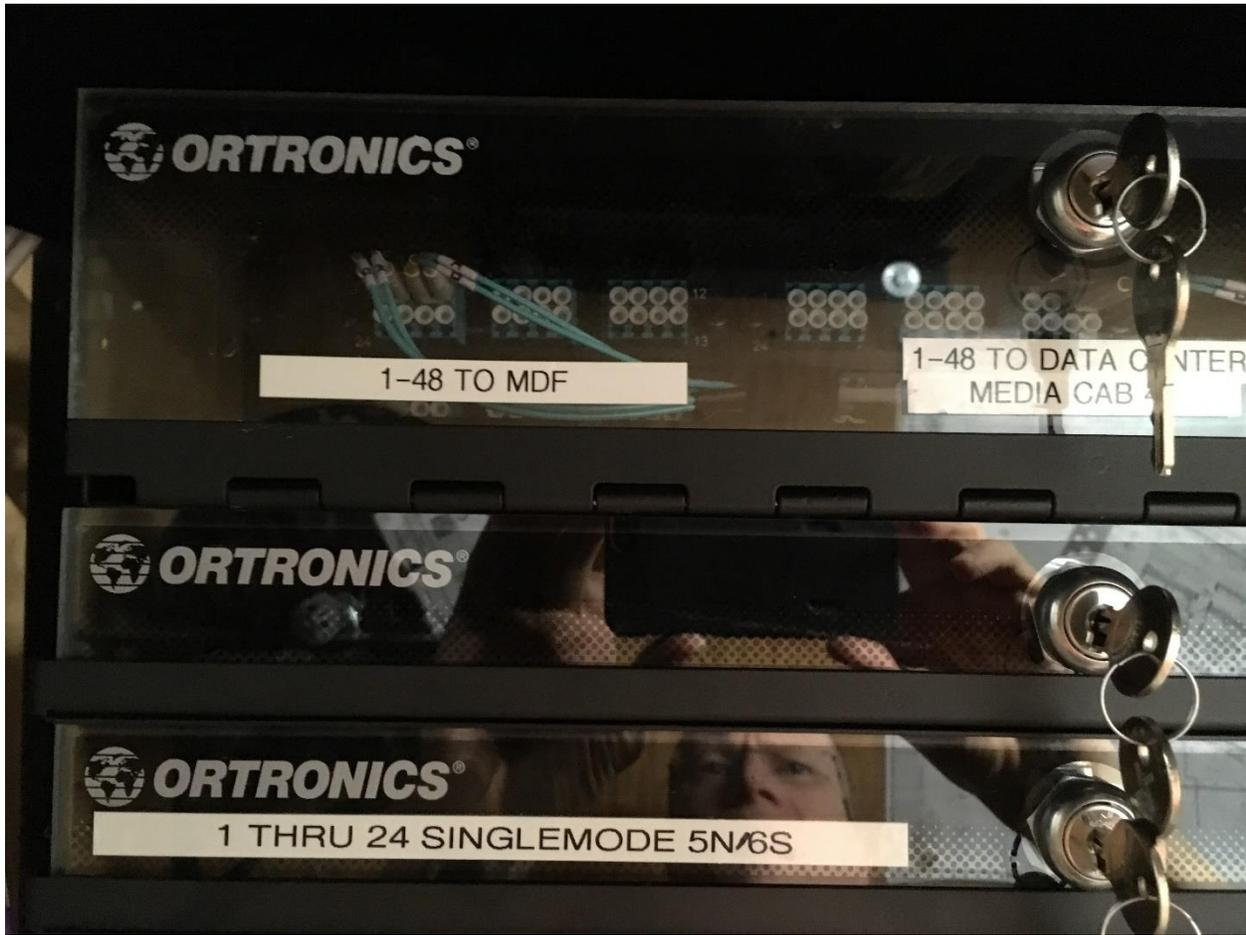
Figure 9: Structured Glass Cabling to MDF
